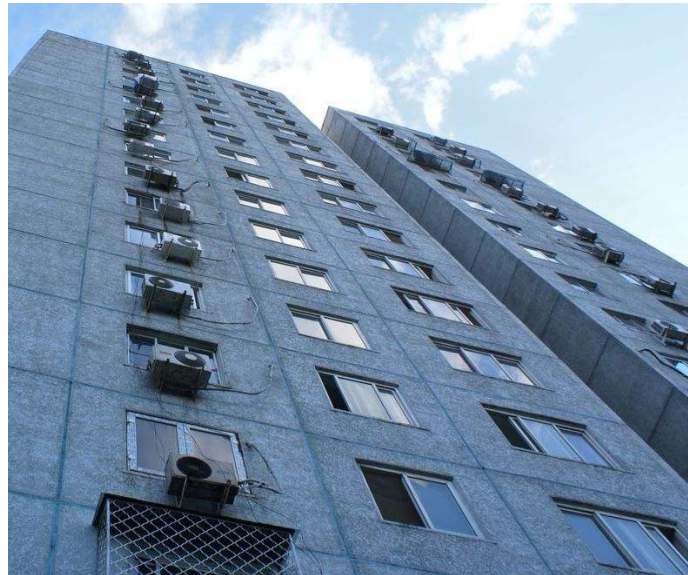
Fig.1. Layout of the air-conditioner condenser for residential buildings
